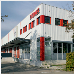
Logistics center in Leinfelden-Echterdingen
