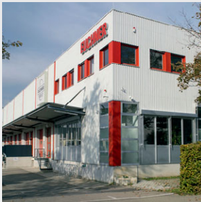
Logistics center in Leinfelden-Echterdingen
