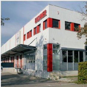
Logistics center in Leinfelden-Echterdingen
