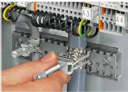
Securing an additional shield clamping saddle.
