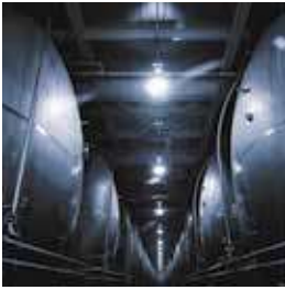
Fill level measurement in tanks
